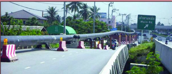
76cm (30") Gas Pipeline – Bangkok, Thailand
