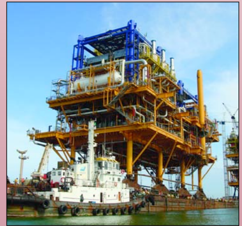
Offshore Platform Topside Module – Swecomex Project, Mexico
